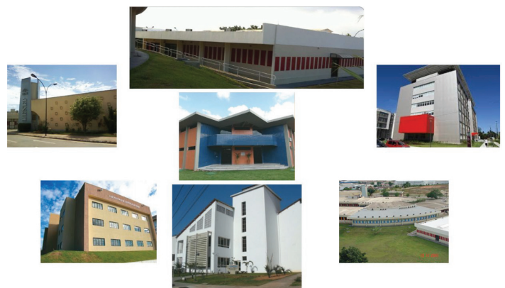
Fig. 4— New facilities for teaching activities and for research laboratories (modified from http://www.anp.gov.br/ ).
